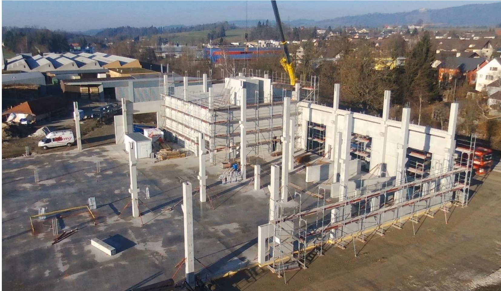
Example – Examples of a industrial building in Wil (Switzerland)
